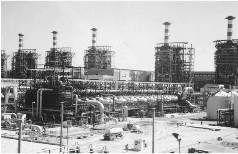
FIGURE 20.6.2 One of the six units of the 346,000 m 3 /day MSF desalination plant Al Taweelah B in Abu Dhabi, United Arab Emirates. (Courtesy of Italimpianti S. p. A.) It is a dual-purpose plant, composed of six identical power and desalination units. Five of the six boilers are seen in the background. The desalination units were in 1996 the largest in the world. They have 17 recovery and 3 reject stages and a performance ratio (PR) of 8.1. The plant also produces 732 MWe of power.
