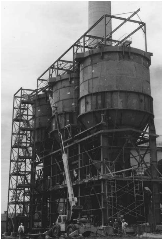
FIGURE 1.5.31 Various pressure vessels. (Photos courtesy Nooter Corp., St. Louis, MO.)
