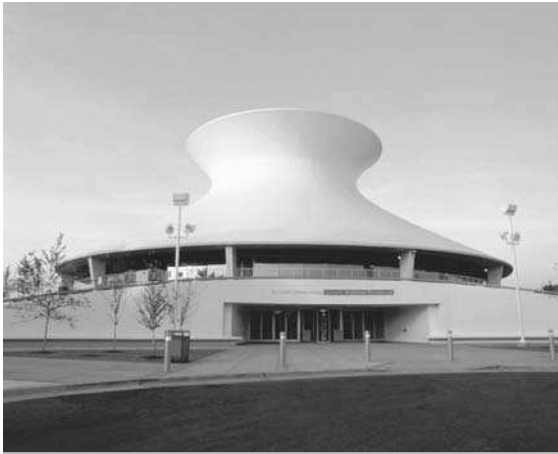
hyperboloid The McDonnell Planetarium in St. Louis is an example of a hyperboloid. Courtesy of the St. Louis Science Center
